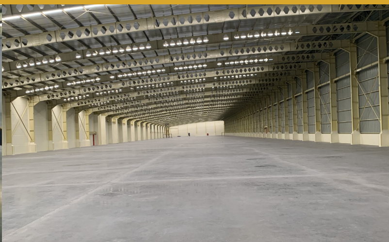
GarudaFood TBK Warehouse, Gresik
